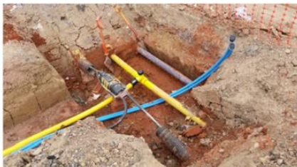
1. Service Pit prepared fully at Stage 1
