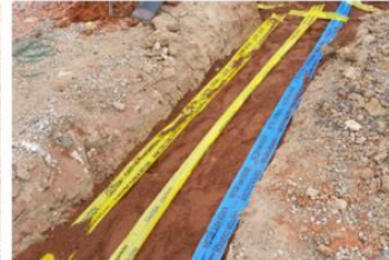
3. All mains correctly backfilled (sand & marker tape)
