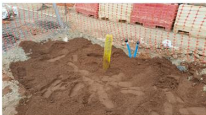
4. Service Pit filled with waste/fill sand
