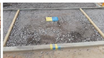
6. Preparing for future gas and water connections with timber bearers and sprayed brick over vertical sleeve
