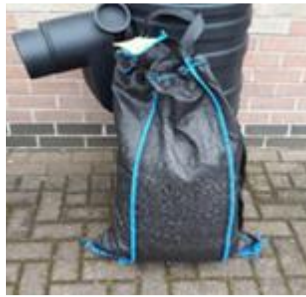
Gully bag silt protection
