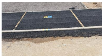
7. Completed Stage 1 footpath with pit ready to be excavated at stage 2 (future connections)
