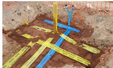
2. Vertical sleeves placed to protect any purge valves (nipples). Loaded with sand and marker tape
