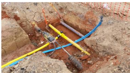
1. Service Pit prepared fully at Stage 1
