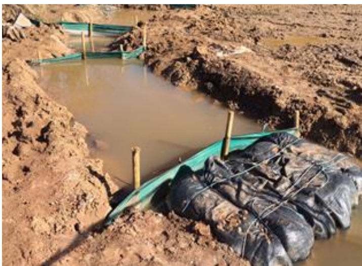
Prevention of silt run off entering water course
