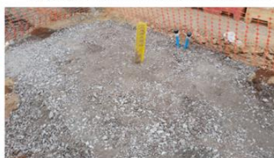
5. Sand then blinded with Type 1 MOT stone
