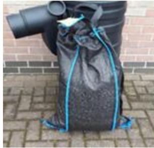
Gully bag silt protection
