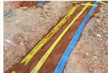
3. All mains correctly backfilled (sand & marker tape)
