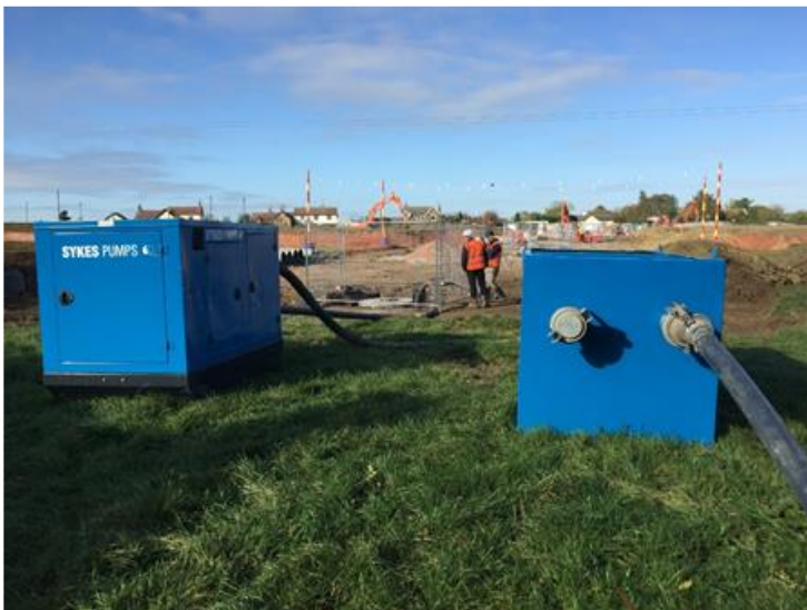
Silt busters fitted on pumps during dewatering operations
