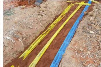
3. All mains correctly backfilled (sand & marker tape)
