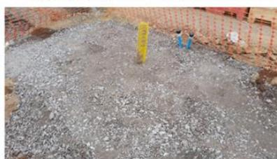
5. Sand then blinded with Type 1 MOT stone
